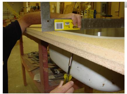
Using a straight edge or square, check the height of the sink rim. It must not be lower than the substrate. Take your time to make sure the sink is level with the substrate or slightly higher than the substrate. You can place thin strips of vertical grade laminate between support board and underside of sink rim to raise the rim where needed. Alternatively use screws through the support boards and tighten as need to adjust sink height.
