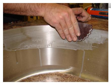
Polishing paste available from Karran along with a maroon 3M Scotch-Brite pad polishes and finishes the sink wall if needed.
