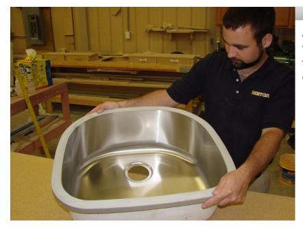
After removing the sink from its box, inspect closely for damage. Check both the rim and the corners of the bowls for any shipping damage. If the sink is damaged, call your Karran distributor immediately.
